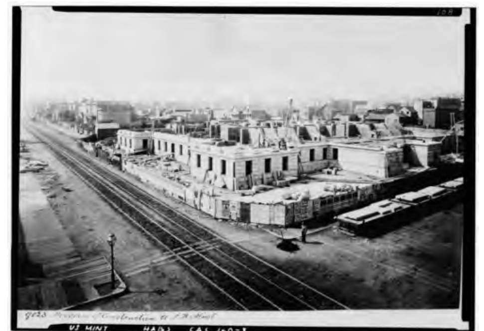
One of a series of Muybridge photos documenting the construction of the San Francisco Mint.
