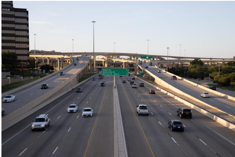
US 75 at High Five with Traffic
